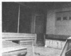
EXTERIOR VIEW OF ENTRANCE DOOR FROM HOUSTON STREET LOADING DOCK
